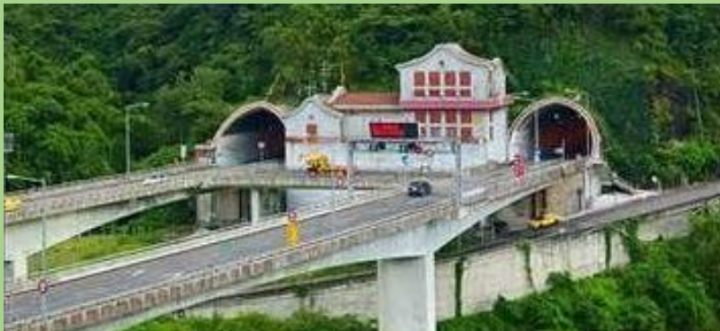
main Hsuehshan Tunnel west portal
