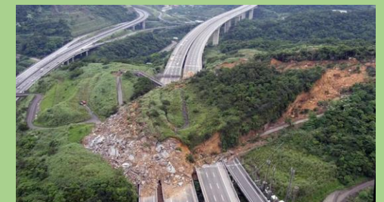
Landslide over a highway
