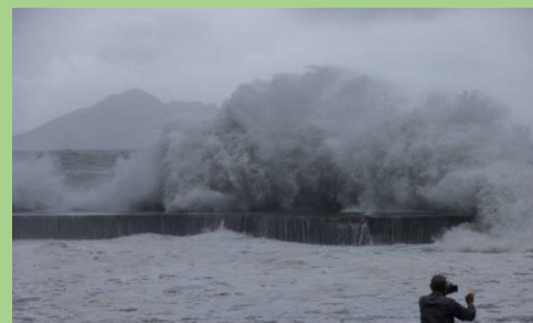
Typhoon surf on breakwater of Toucheng Harbor
