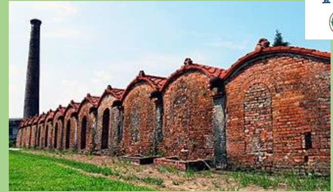
Historic Chen He Cheng Kiln Factory, (brick works) built 1831
